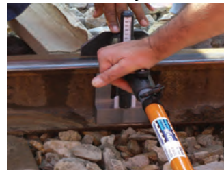
Measuring the height to determine packer size
