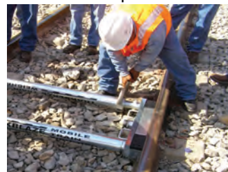
Inserting the MTW into the track and expanding the system via the threaded support poles
