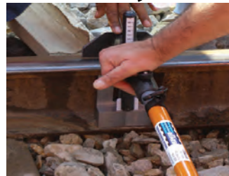
Measuring the height to determine packer size
