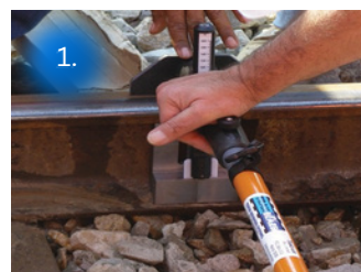
1. Measuring the height to determine packer size
