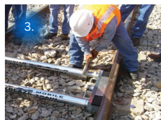
3. Inserting the MTW into the track and expanding the system via the threaded support poles
