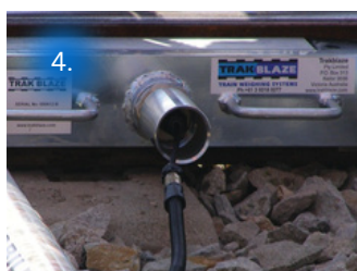
4. Connecting the cables, wireless option also available
