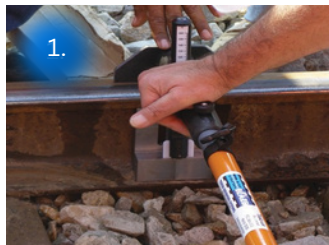
1. Measuring the height to determine packer size
