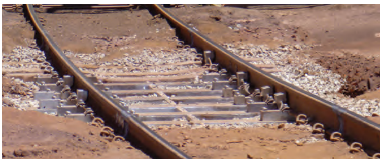
Installation of INFINITY 'LS' weighing system in curved track
